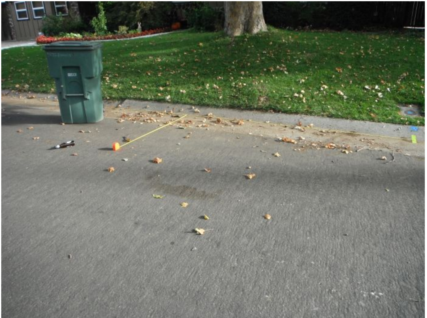
Photo 2: Station line measurements taken perpendicular from the tape measure to a screw driver.
